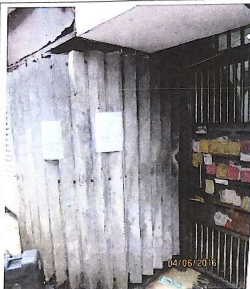
G/F staircase, 33 Kai Ming Street
