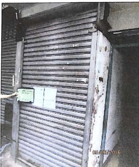
G/F staircase, 37 Kai Ming Street
