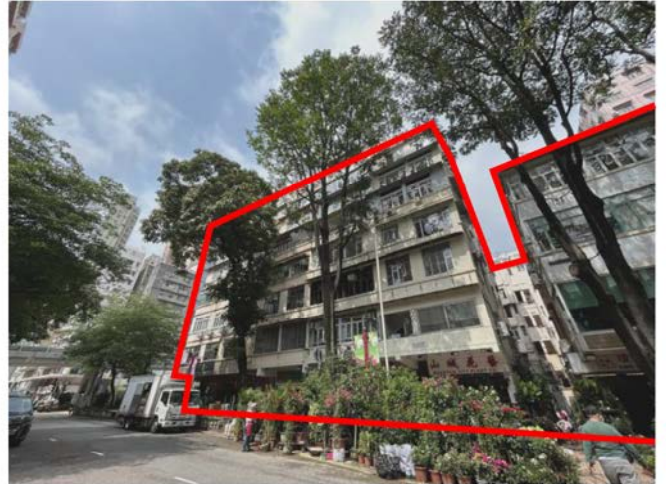
VIEW 2: BUILDINGS WITHIN SCHEME AREA ALONG SAI YEE STREET
