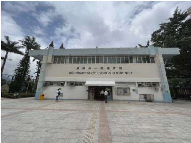
VIEW 8: BOUNDARY STREET SPORTS CENTRE NO.1
