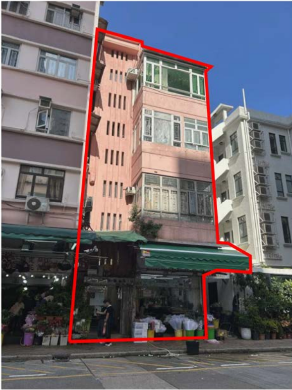
VIEW 5: A BUILDING WITHIN SCHEME AREA ALONG YUEN NGAI STREET
