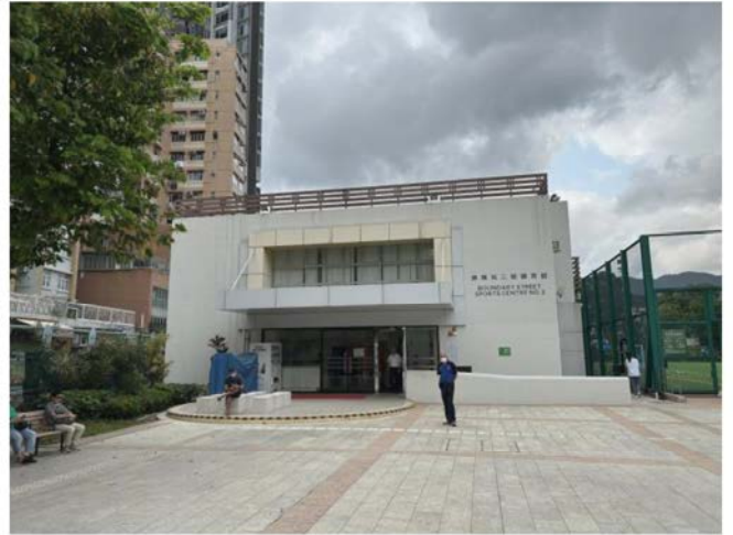
VIEW 9: BOUNDARY STREET SPORTS CENTRE NO.2
