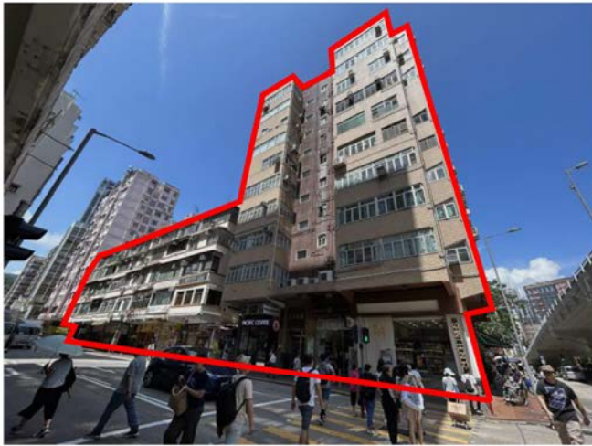
VIEW 1: BUILDINGS WITHIN SCHEME AREA ALONG FA YUEN STREET
