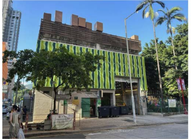
VIEW 14: SAI YEE STREET (FLOWER MARKET ROAD) REFUSE COLLECTION POINT-CUM-SAI YEE STREET PUBLIC TOILET
