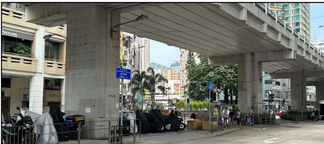
Figure 8 Space beneath the flyover along Prince Edward Road West
